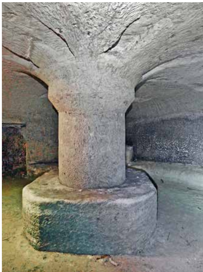
Willoughby House: the massive pillar in the centre of the largest of the circular cellars. Photo Tim Wellburn
